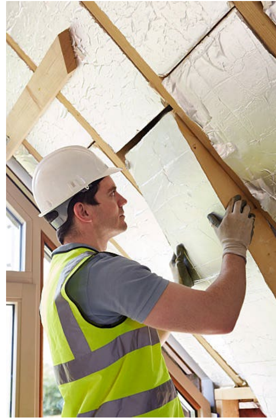
Home renovation or repairs
